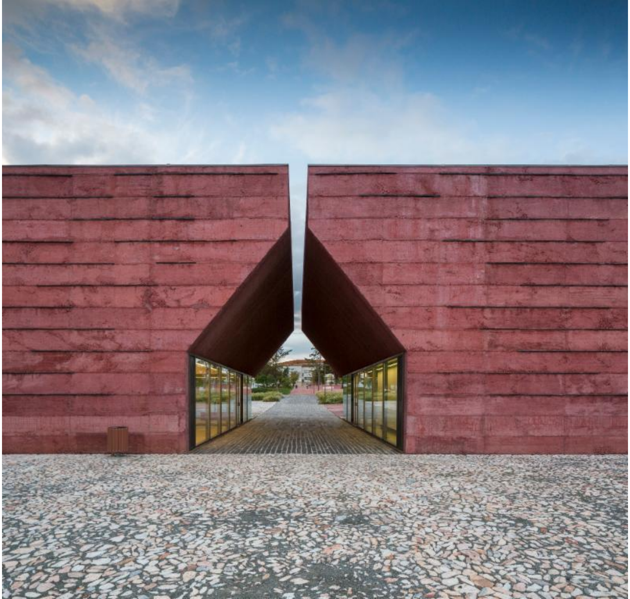
Photo courtesy of Gonçalo Byrne, photo credit to Fernando Guerra.
