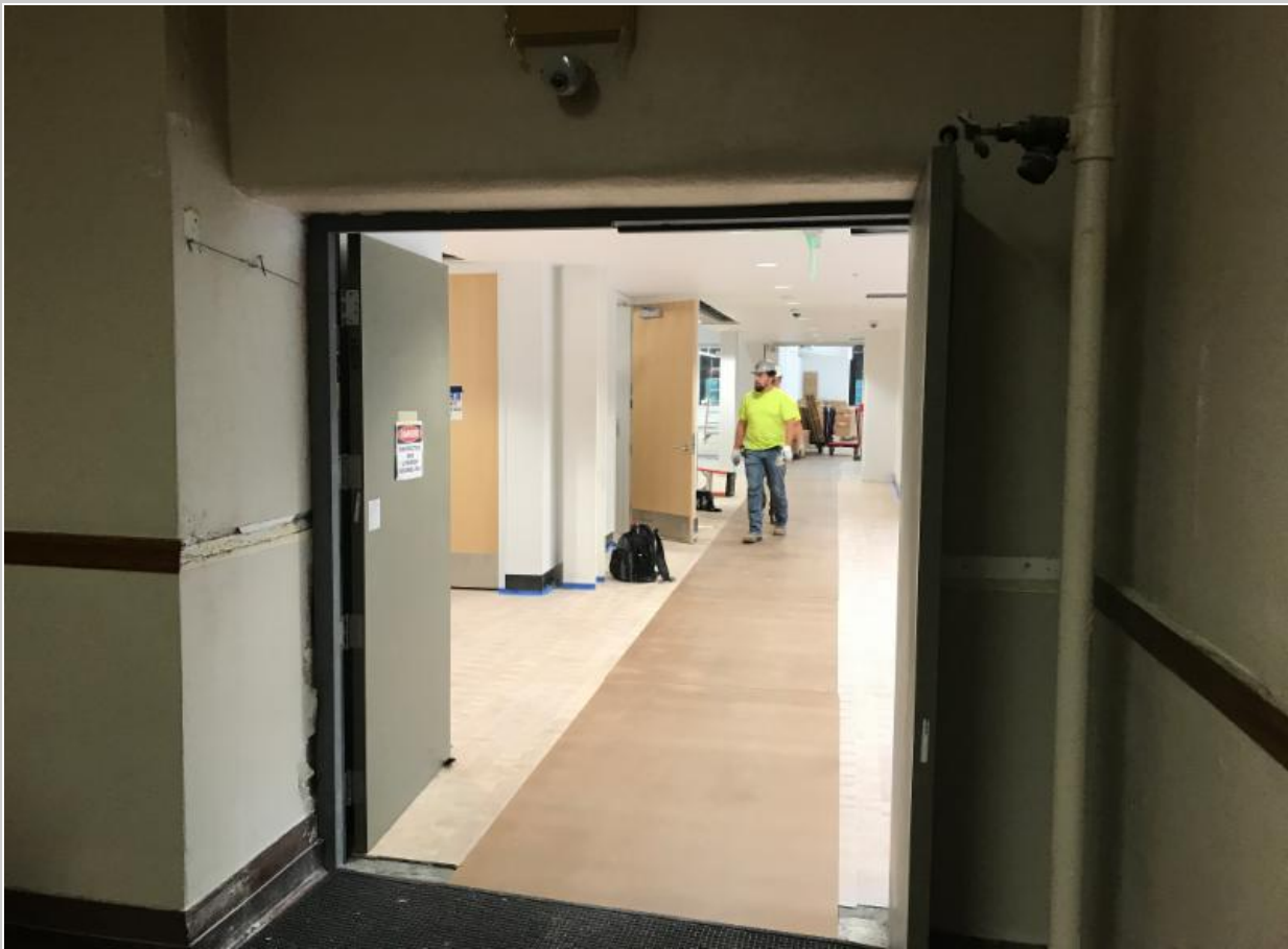
A sneak peak down the newly renovated first floor hallway
