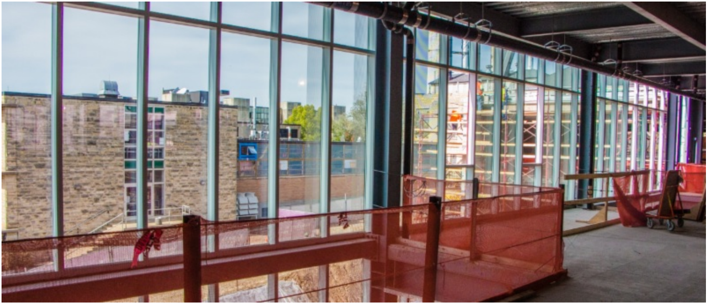
Windows going in on the west side of the new construction
